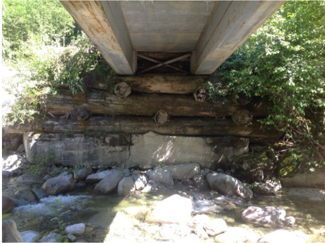
Left Bank Abutment when facing downstream
