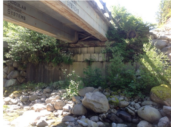
Right Bank Abutment when facing downstream
