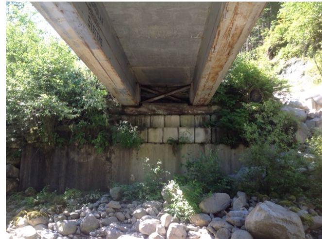
Right Bank Abutment when facing downstream
